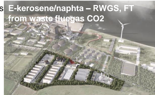
E-kerosene/naphta – RWGS, FT from waste fluegas CO2 Copenhagen Infrastructure Partners, Reno Nord, Aalborg Forsyning, Aalborg, Denmark 80.000 tons e-kerosene/y + 17.000 e-naphta/y (2027)
