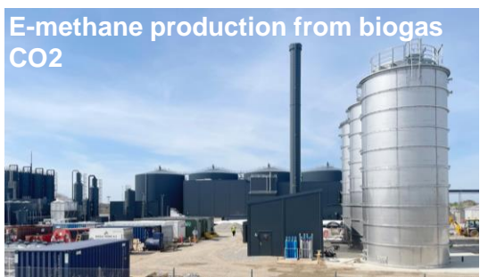
E-methane production from biogas CO2 Nature Energy, Biogasclean, Andel, SDU Glansager, near Sønderborg, Denmark Kick-off (3rd Nov. 2023), 13 million m3/year (2024)
